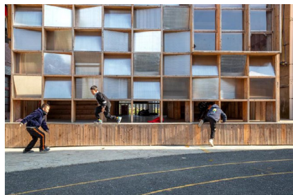
↑ Figure 13 + 14: Repurpose - (top) slums in Indonesia using patches of discarded materials, (bottom) library project using small pieces of polycarbonate for the facade
