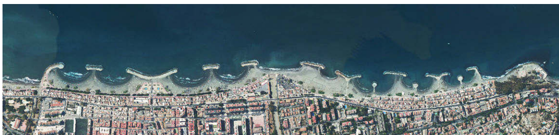
Figure 10.41: Real-life example: tomolos behind emerged (i.e. having their crests above MSL) offshore breakwaters in Malaga, Spain. Photo from SCNE ('Credits' on page 579).
