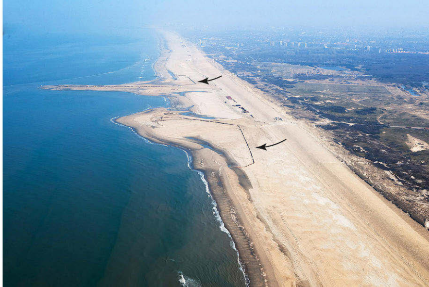
Figure 10.32: Beach suppletion during construction of the Sand Engine using pipelines (indicated by the black arrows) that cross the breaker zone in March 2011. From Rijkswaterstaat ('Credits' on page 579).
