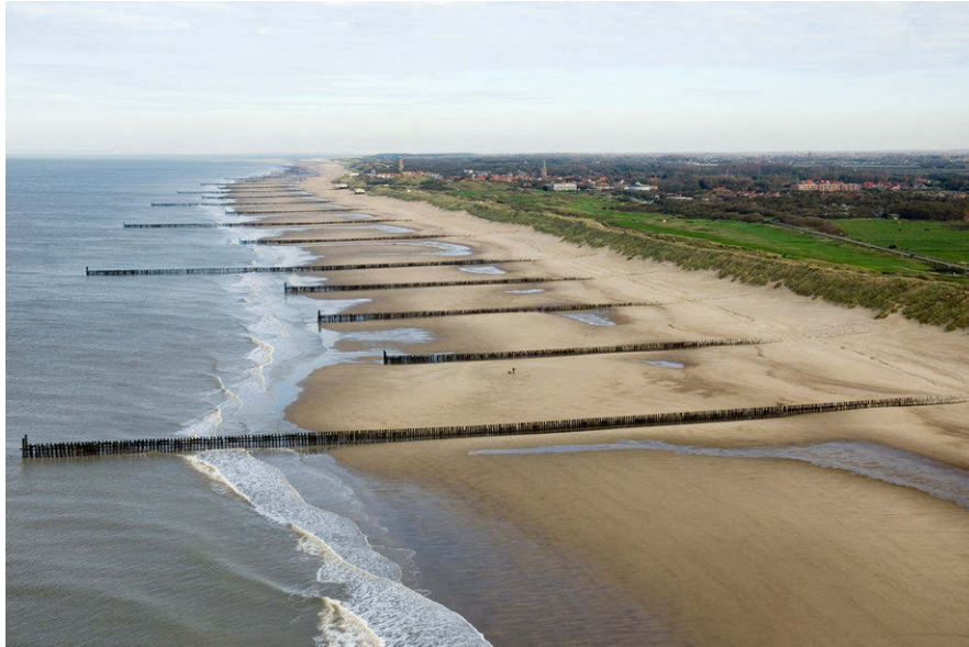
Figure 10.13: Groynes on the Dutch southwestern delta coast, near Domburg, in November 2005. Photo from Rijkswaterstaat ('Credits' on page 579).
