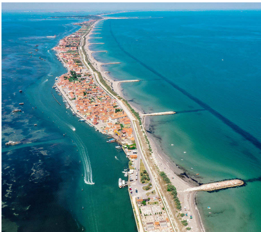
Figure 10.40: Submerged breakwater serving to perch the beach nourishment at the Pellestrina barrier island, in Venice, Italy. On the left side the Venetian Lagoon and on the right side the Adriatic Sea. Photo by Ni_Giri ('Credits' on page 579).
