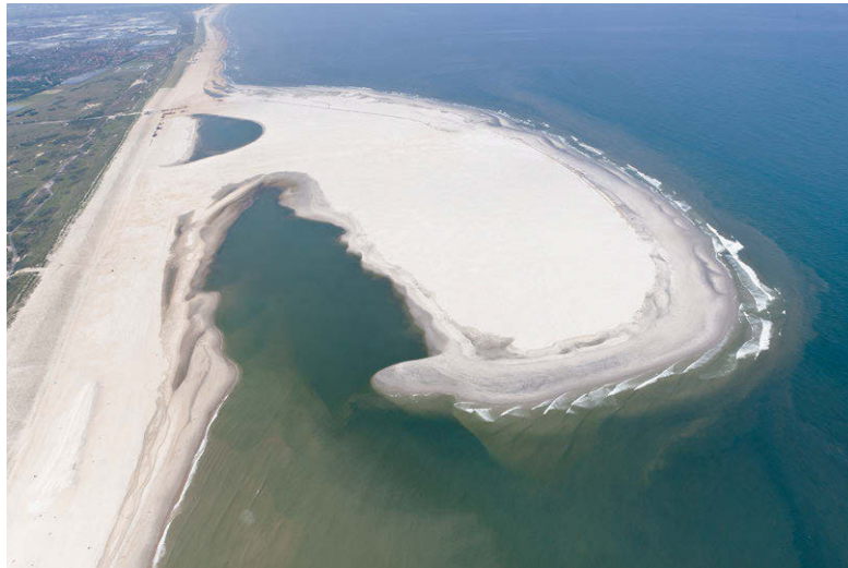
(a) just after completion in 2011
