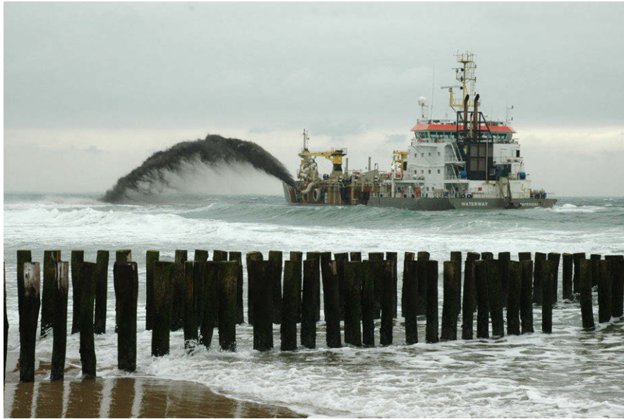
Figure 10.33: Shoreface nourishment at the Dutch coast through rainbowing in September 2005. From Rijkswaterstaat ('Credits' on page 579).
