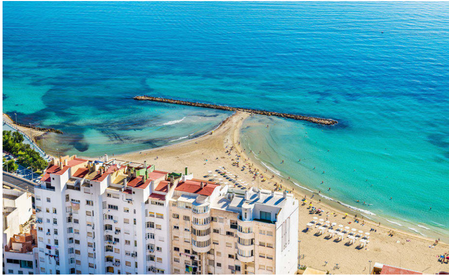
Figure 8.21: Tombolo formed behind a detached breakwater in Alicante, Spain. Photo by Leonid Andronov ('Credits' on page 579).
