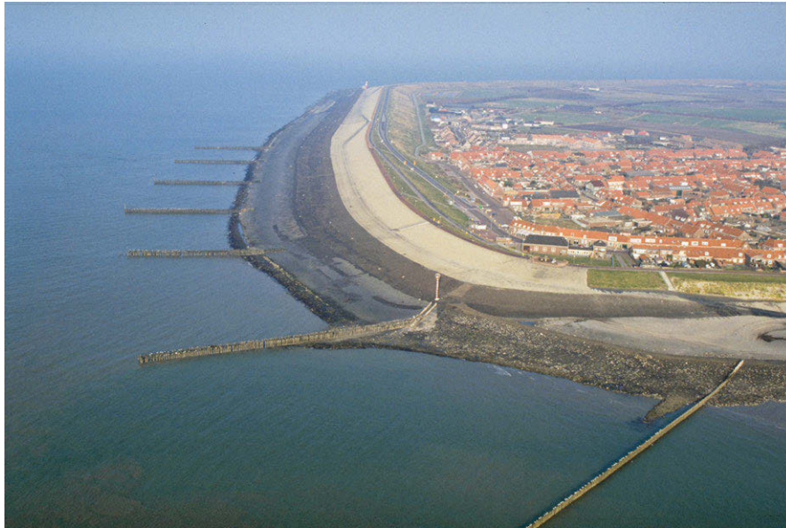
Figure 10.28: Sea dike, Westkapelle, the Netherlands, in June 1993. From Rijkswaterstaat ('Credits' on page 579).
