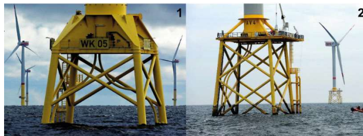
Figure 1 – Jacket types without (Type 1, Left) and with (Type 2, Right) waterline crossing braces
