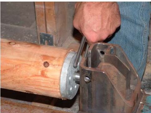
fixing the prestress in the wood
