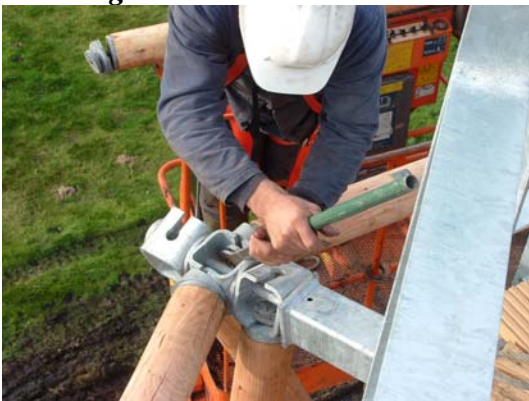
Tightening of a locking disk inside a chaining block
