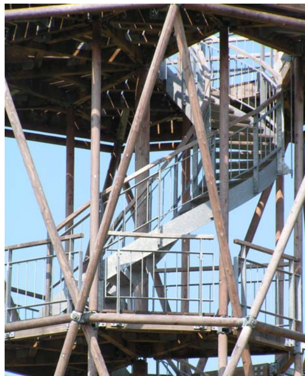
Home grown small diameter larch beams. Central steel stairway
