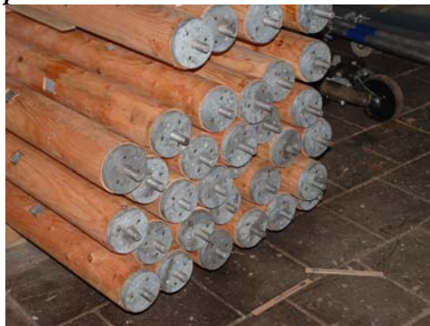
beams ready for assembly in the tower
