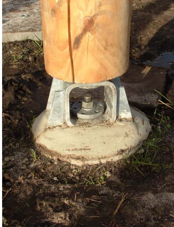
Foundation detail central column
