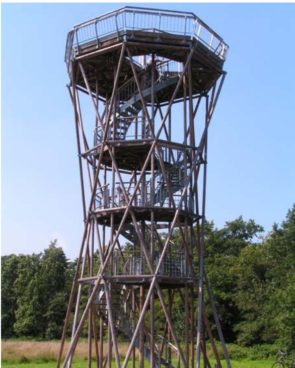
Viewing platform Holmers Halkenbroek, Drenthe
