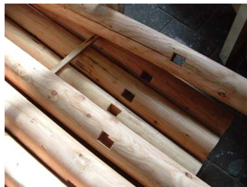
milled anchor block chambers
