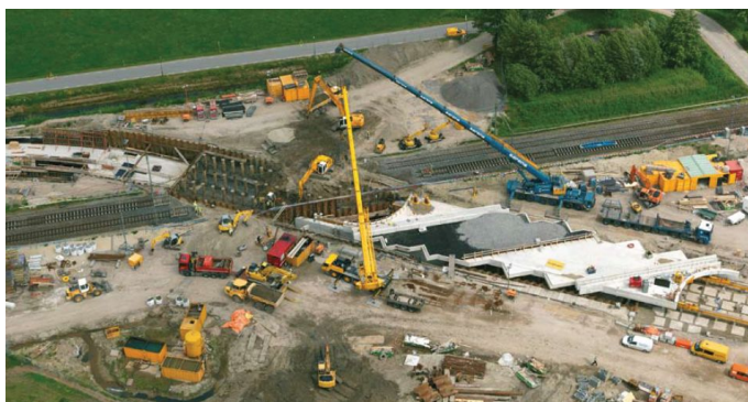
Figure 2.7: Method of the inserted deck applied at the underpass Fortweg between Utrecht and Houten [15]
