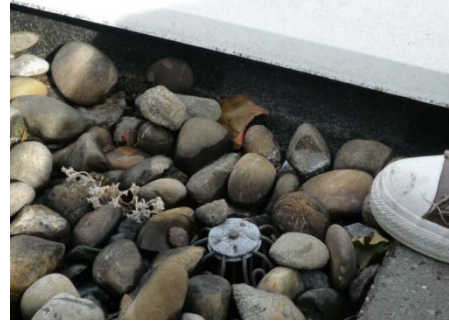
Figure 24: Roof of elevator shaft NOT in shadow of high rise
