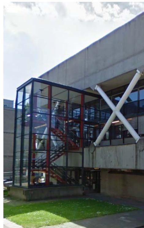
Figure 13: Stairway Faculty of Civil engineering
