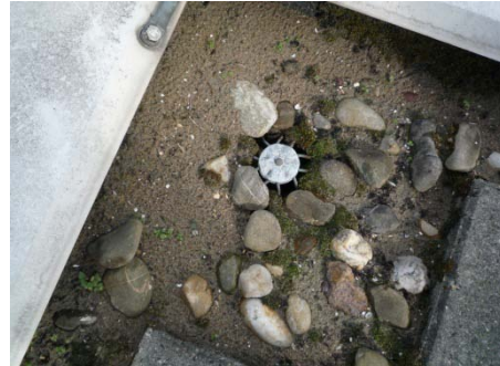
Figure 25: Roof of elevator shaft IN shadow of high rise
