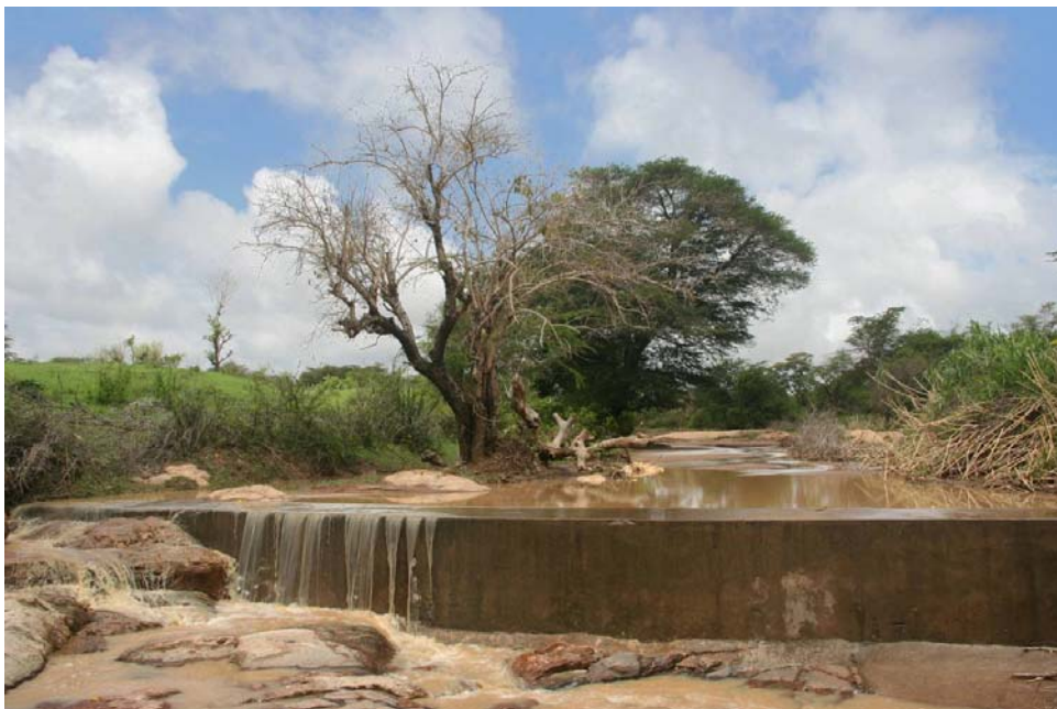
Figure 1.3. Sand storage dam in Kitui (Source: Borst and de Haas)
