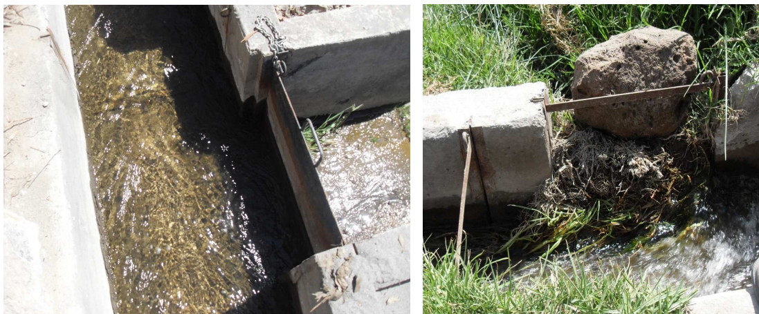
Figure 14: Lateral gates
