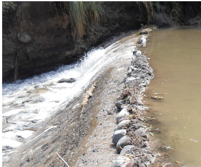
Figure 13: Dike of concrete in Bajo Yarabamba
