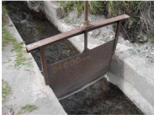
Picture 1: Head gate of Alto Quequeña
