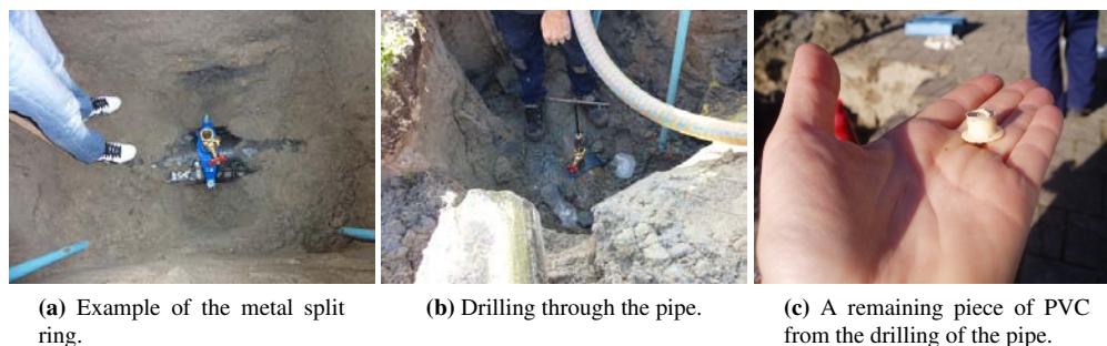
Figure A.14: Boring the opening for a sensor S1.
