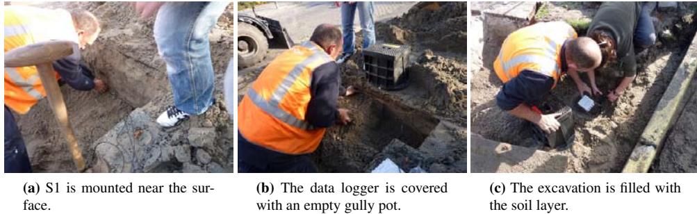
Figure A.16: Earth works at location 2.
