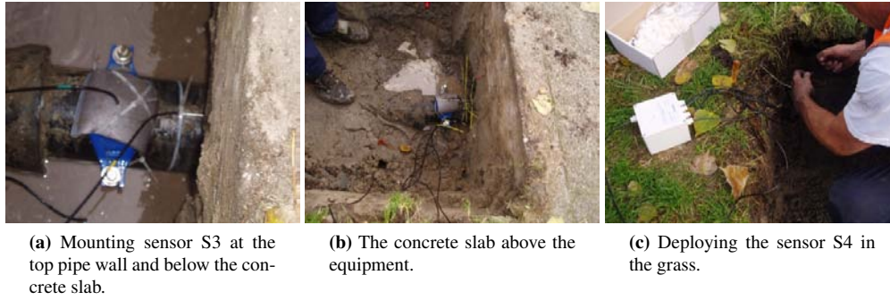
Figure A.19: Sensors set-up in the soil at location 4.
