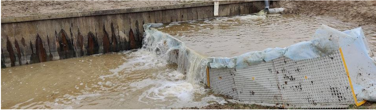
Figure 8: overtopped H-wall (own work)
