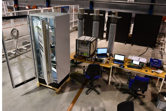
150kV LPIT setup at KEMA Labs
