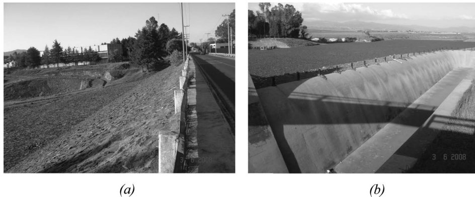
Figure 1. Recent photographs of the José Antonio Alzate dam (San Bernabé). (a) Downstream slope (embankment). (b) Reservoir and spillway.
