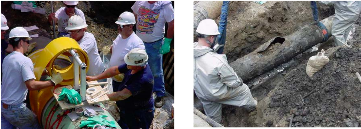
Figure 1-3: clock spring installation (left), gas pipeline excavation (right)
