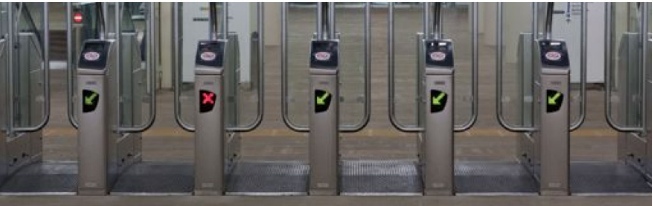
Figure 12: A line of gates in Rotterdam Central metro station, a clear payment border.
