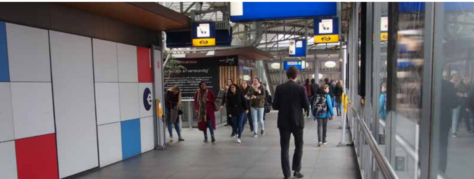
Figure 36: Rear side of Den Bosch station. On one side, the sign could not be hung above the OV-chipkaart post, due to limited height. Moreover, this sign is one-sided.
