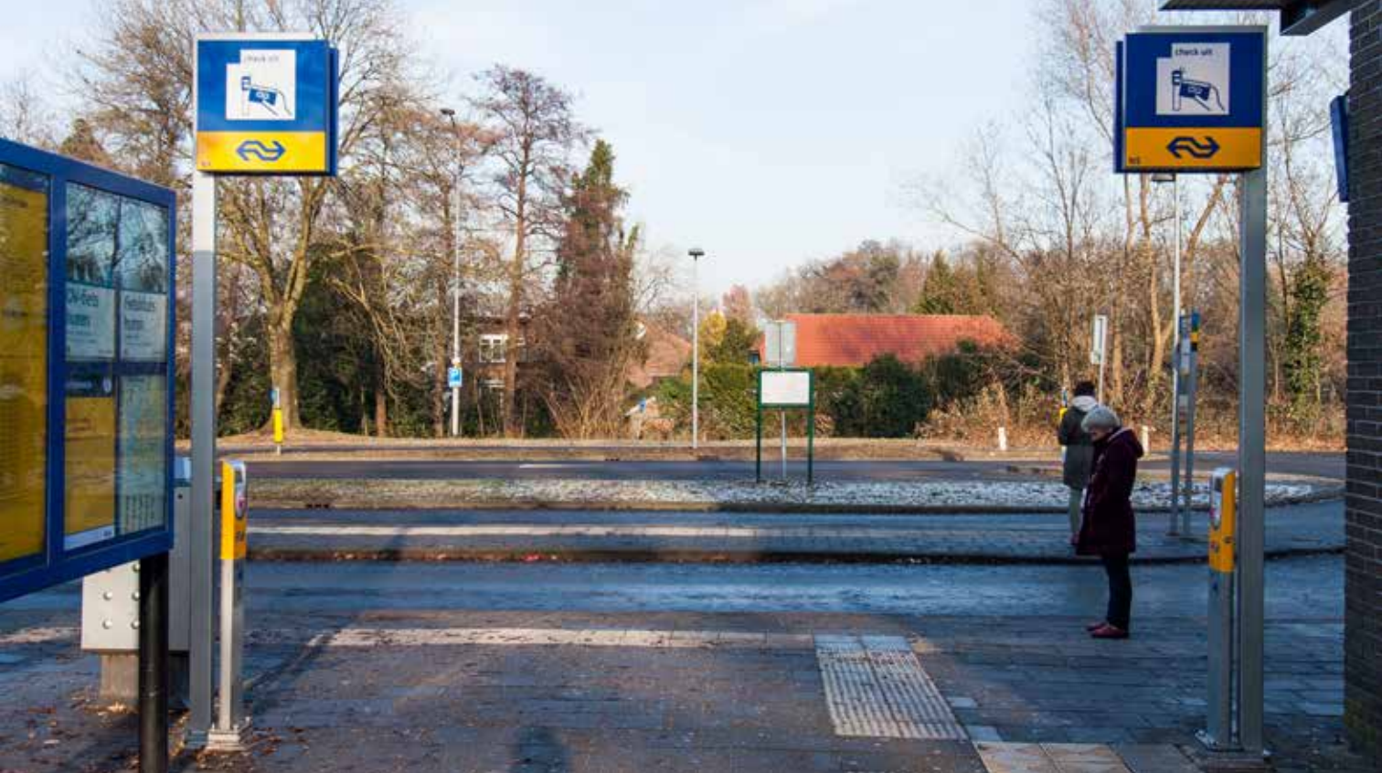
Figure 39: The installation on the side of the bus stops.
