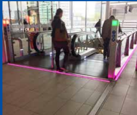
LED-line along all access points from the hall to the platform (Utrecht CS).
