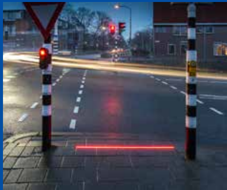
Halt line on the pedestrian crossing: intended to draw attention to the signal of the traffic light while using a telephone.
