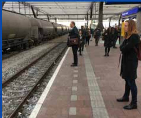
Three markings on the platform: end of the platform (solid line), safe zone ('dotted line'), guide line.
