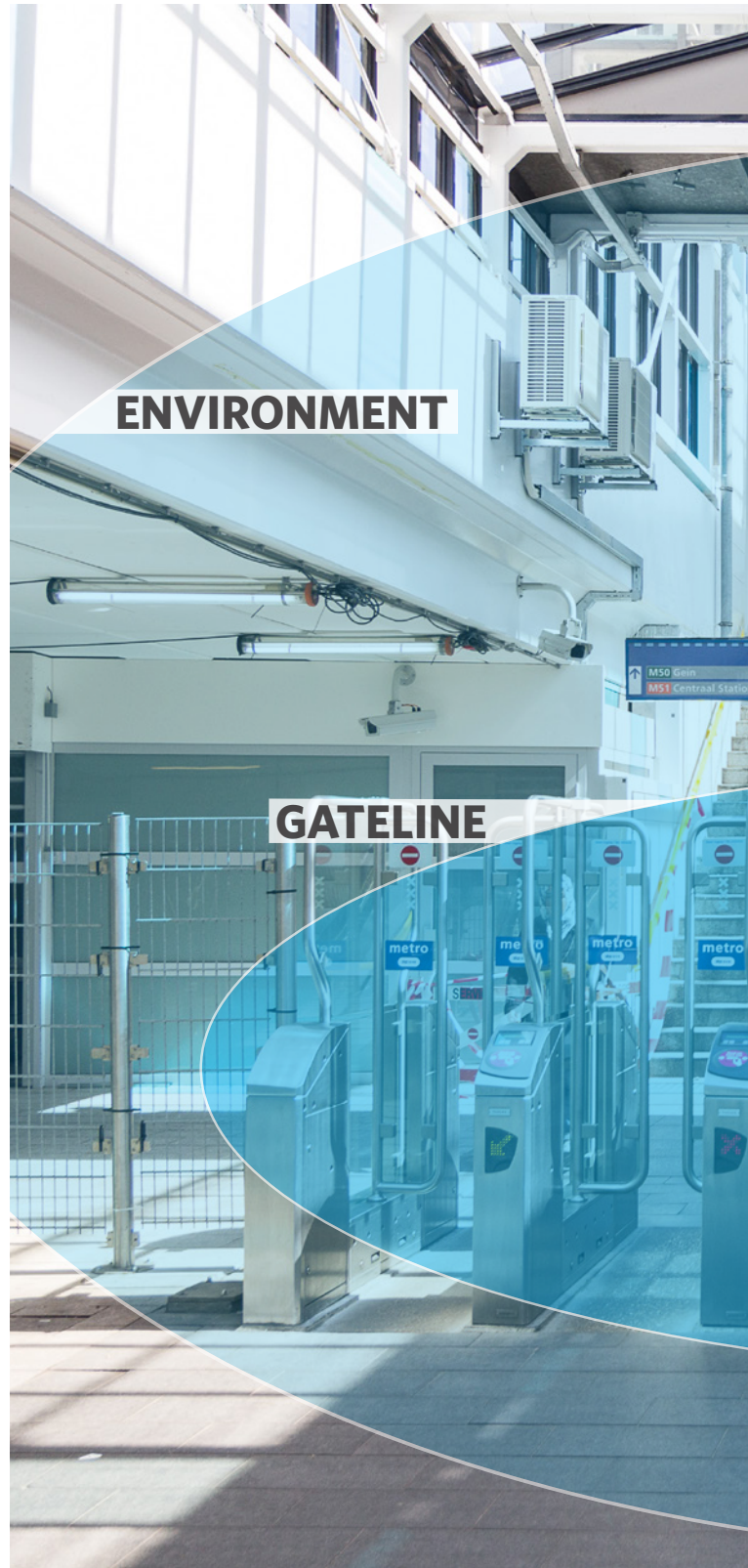
Figure 22. Interaction with closed payment borders takes place on four levels: 1) user interface, 2) gate, 3) gateline and 4) environment
