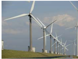
Strain and vibration monitoring
