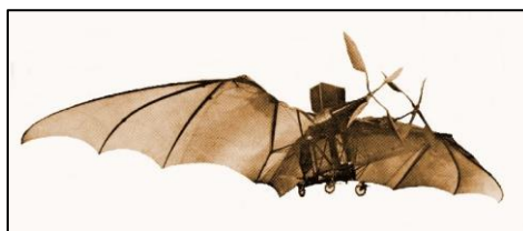
Figure 3.4 – The Éole III, a bat-like flying wing design by Clément Ader which crashed at the first flight, picture from [13]
