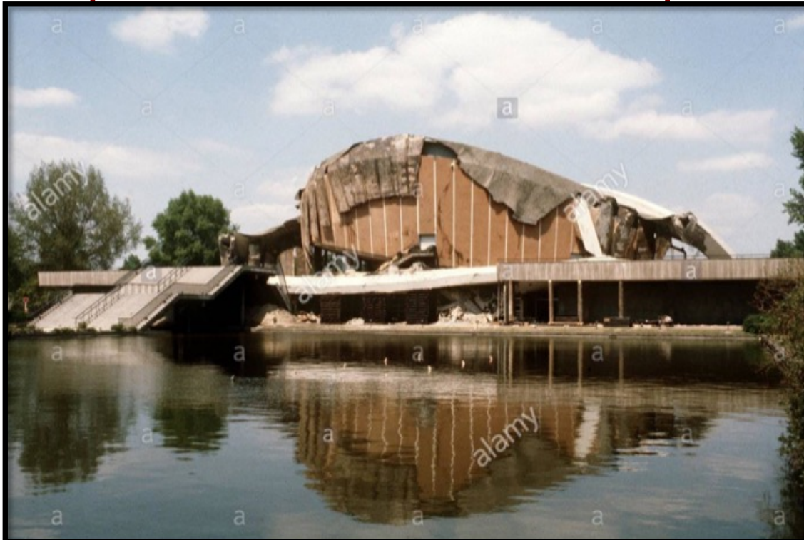
Hydrogen intake causing collapse of roof
