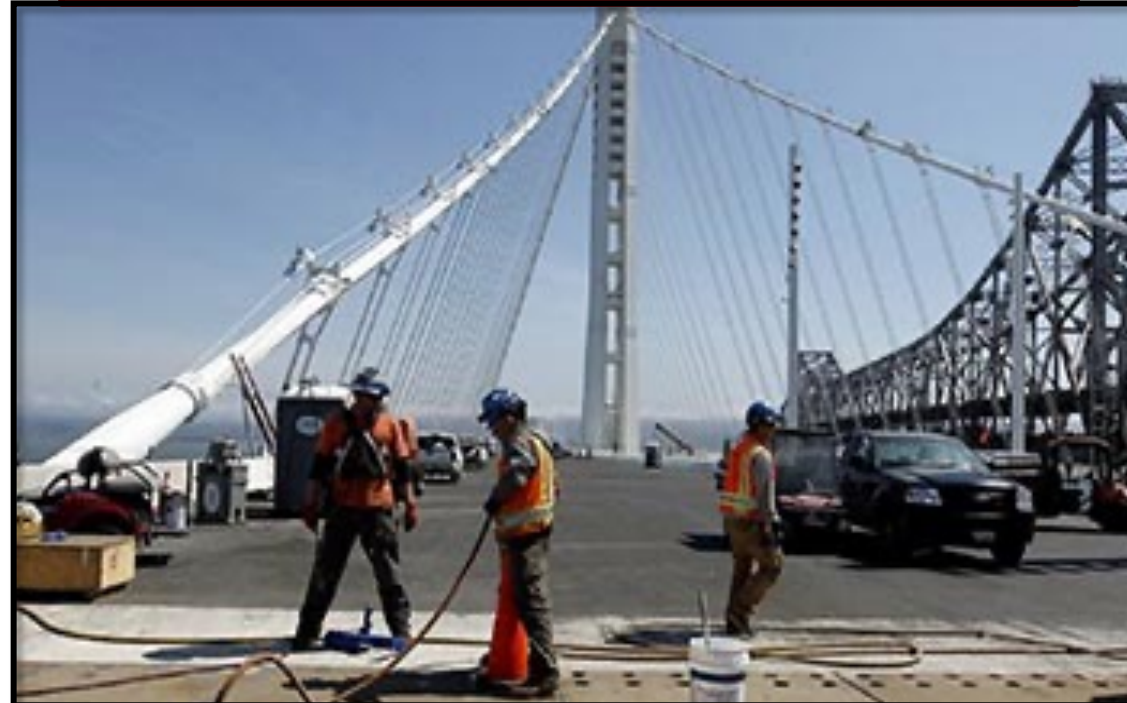
Brittle bolts and cracking due to hydrogen contamination
