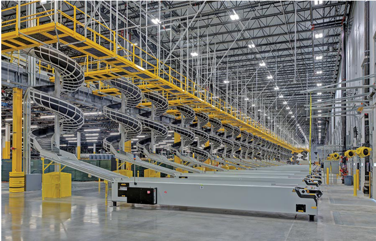
Amazon Fulfillment Center, Las Vegas © Layton Construction
