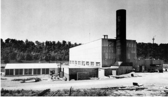
Figure 1.2: The ARE building at Oak Ridge National Laboratory was first used for the Aircraft Reactor Experiment and later for the Molten Salt Reactor Experiment.
