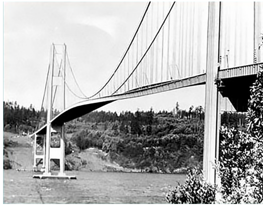
Figure 1.6: The bridge over the Tacoma Narrows before its collapse: the frequency of oscillation of the bridge modulated the shedding frequency with which vortices of air were being shed downstream. This led to a self-excitation which eventually led to the collapse of the structure even though the frequency of oscillations did not match the natural frequency of the bridge. Adopted from [29].
