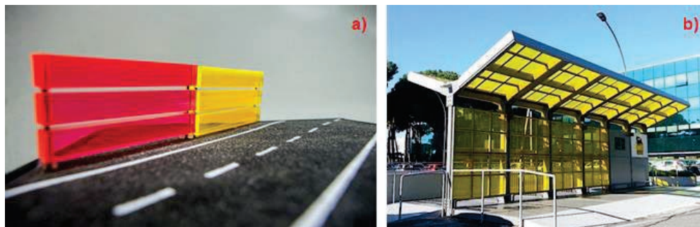
Figure 1.5 Two examples of LSC systems applied in sustainable applications. a) scale model of the Heijmans N.V.. solar noise barrier [33] and b) the Eni bus shelter in Rome that serves as a charging station for electronic bikes. [31]
