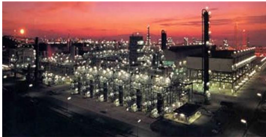
Figure 1.2: Shell's Pearl GTL plant in Qatar [22].
