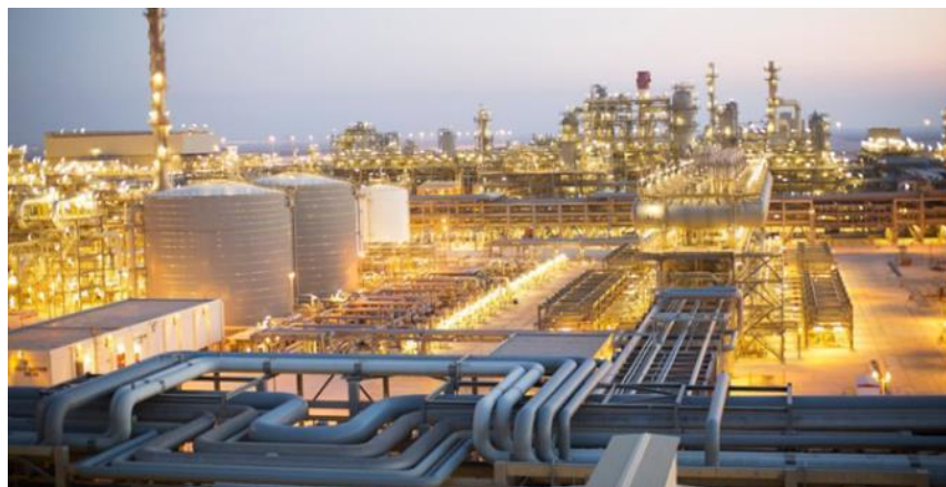
Figure 1.3: Shell's GTL plant in Bintulu, Malaysia [23].
