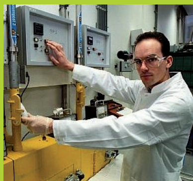
Figure 10: Pneumatically operated small-target irradiation facilities. The photograph shows the PE rabbit loaded into the inlet of the pneumatically operated transport system (to and from the irradiation position).
