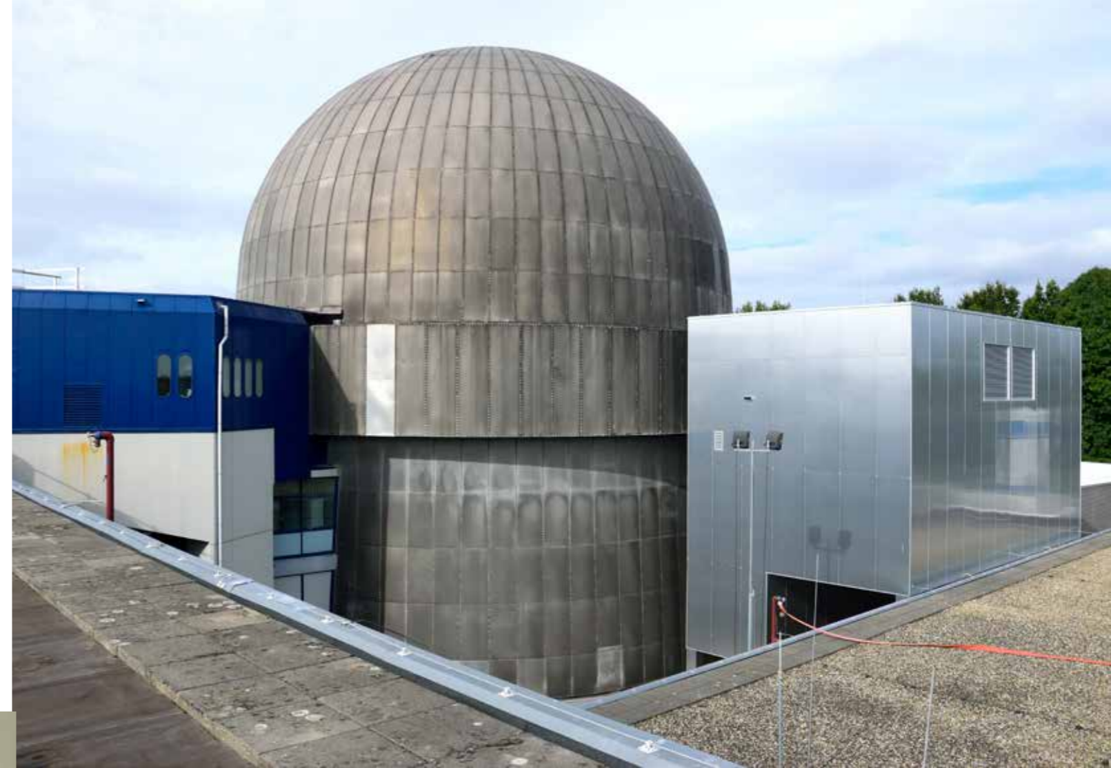
Photo: The reactor hall and the CNS-Utility building.
