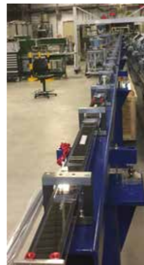
Photo right: New 20 m long neutron guide to transport the neutrons from the cold-neutron source to the neutron reflectometer ROG.
