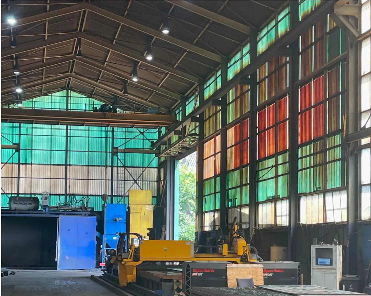
industrial warehouse located in the 'Waterdriehoek' (Hermkens, 2023)
