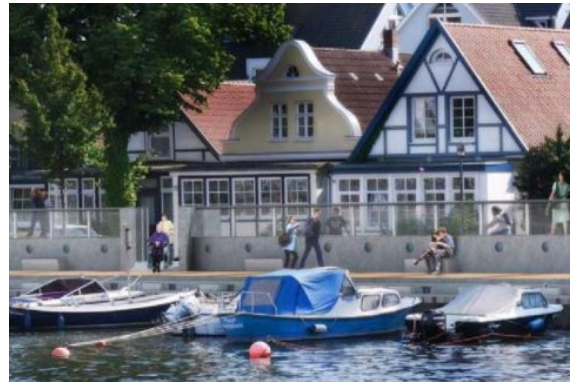
(b) An impression of a glass storm flood protection barrier in Warnemünde (Heyder, Frank en Paulu, Franziska, 2014)
