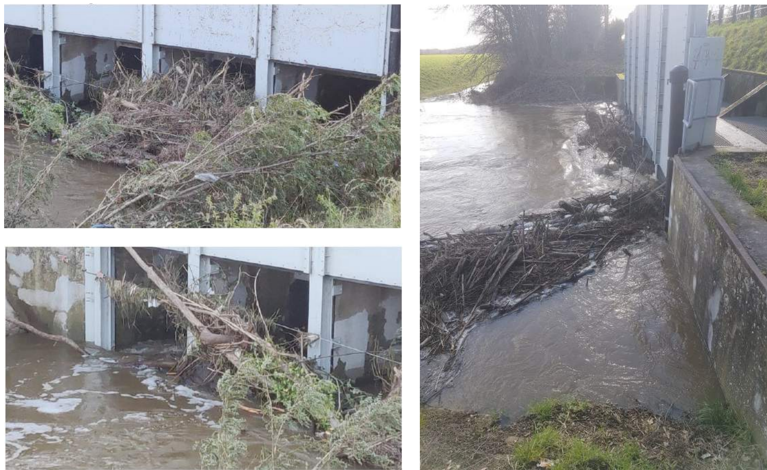
Inverted syphon in Bunde (Limburg, NL), where the River Geul crosses the Juliana Canal
