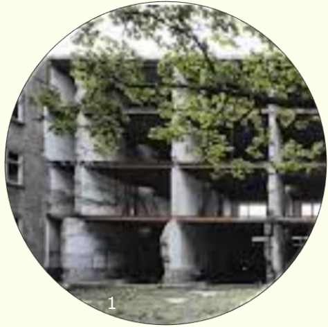
Long term - construction (1930s)
