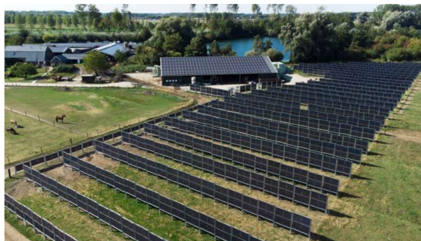
Bifacial agri-PV (Solar park Stal den Heuvel Culemborg, NL)
