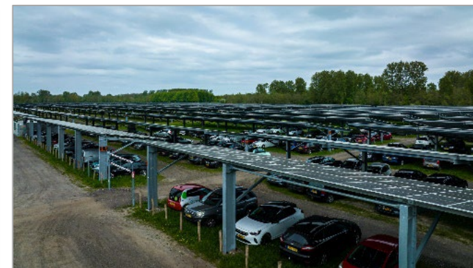
Solar carport Lowlands, Biddinghuizen, NL (photo: Solarfields)
