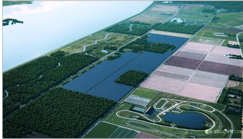
Solar park Dorhout Mees, Biddinghuizen, NL (144 MWp; Solarfields, 2022)
