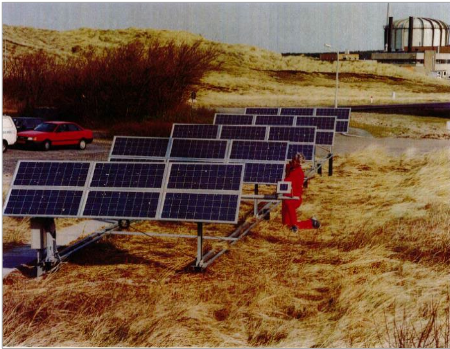
Grid-connected system, Petten, NL (1 kWp; ECN, 1989)
