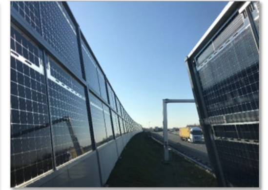
Solar Highways, Uden, NL
