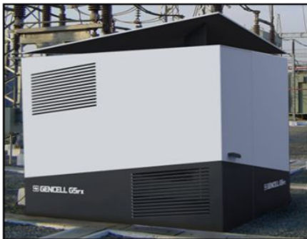
Ammonia fuel cell Electricity from Ammonia-Water
