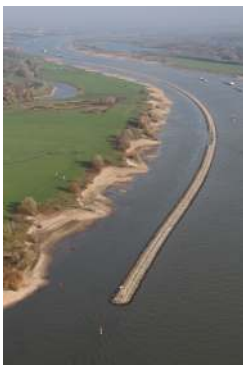
Longitudinal training dam as a river intervention along the river Waal, The Netherlands (source: Rijkswaterstaat).
