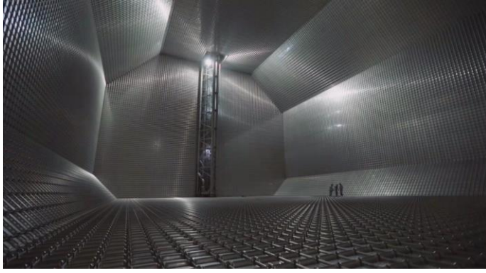
Figure 1. The interior of a Mark III LNG membrane tank.
