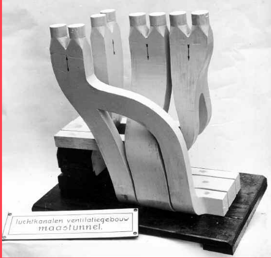
• Airchannels ventilationbuilding • Maastunnel
