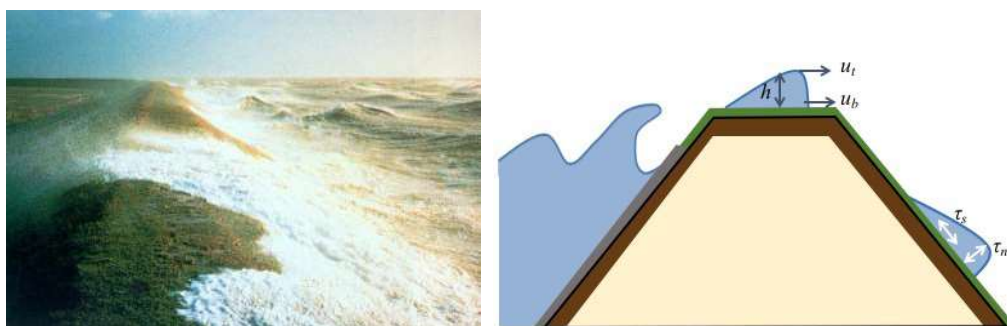
Figure 1: Waves approach the dike and break on the seaward dike slope. The broken waves run up the dike, overtop the crest and then run down along the landward slope. Left: photograph of grass covered dike during wave overtopping [5] (Picture courtesy: HR Wallingford). Right: Schematization of wave overtopping on a grass-covered dike. The overtopping flow has a layer thickness h , the flow velocity near the bed u_b and the flow velocity in the top layer u_t . Typical layer thickness and velocities range between 1-50 cm and 1-10 m/s respectively. The waves pull on the grass cover with a shear stress \tau_s parallel to the dike surface and a normal stress \tau_n perpendicular to the dike surface (figure adapter after [4]).
