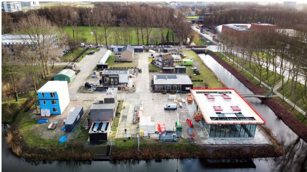
Aerial photo of the Green Village. 10
