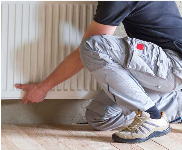
Replacing existing radiators with LT Radiators
