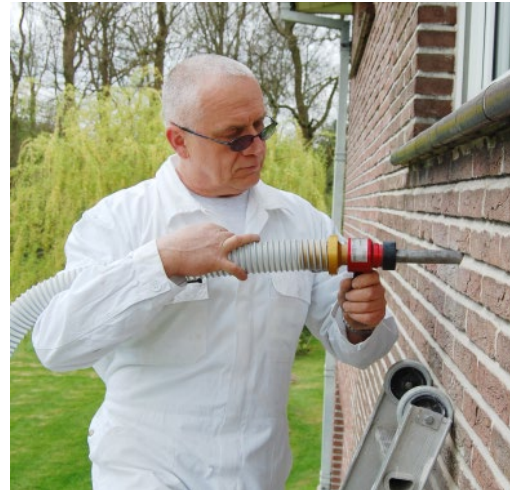
Post insulation of cavity wall
