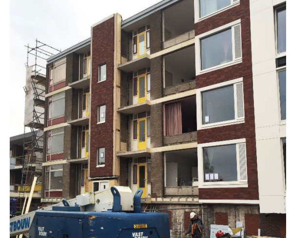
Replacement of building envelope
