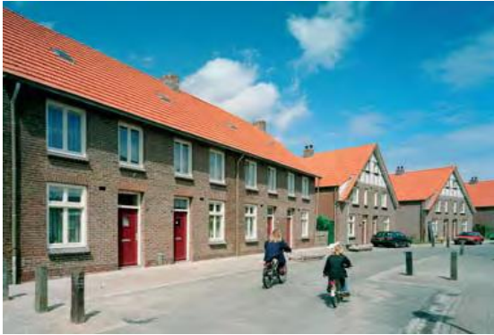
Terraced house archetype built between 1945-1975.
