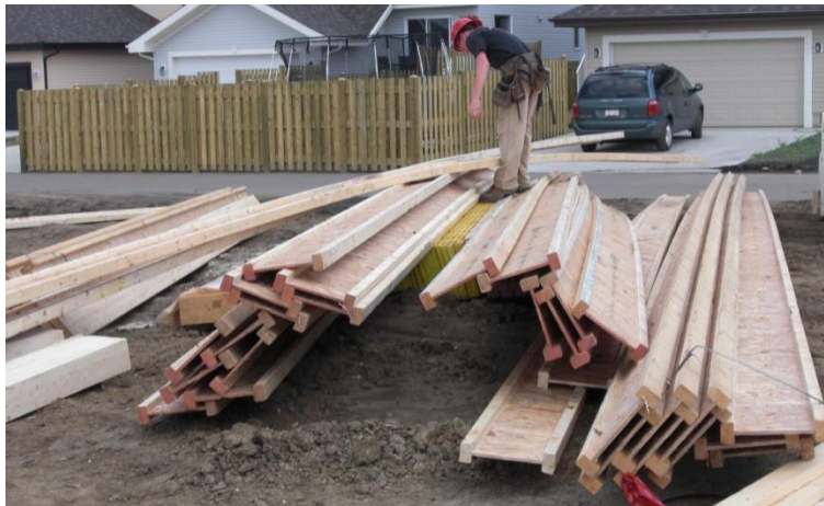
Figure 4: Floor joist package
