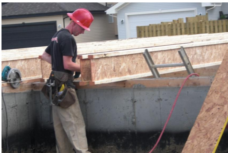
Figure 5: Joist being cut to correct length
