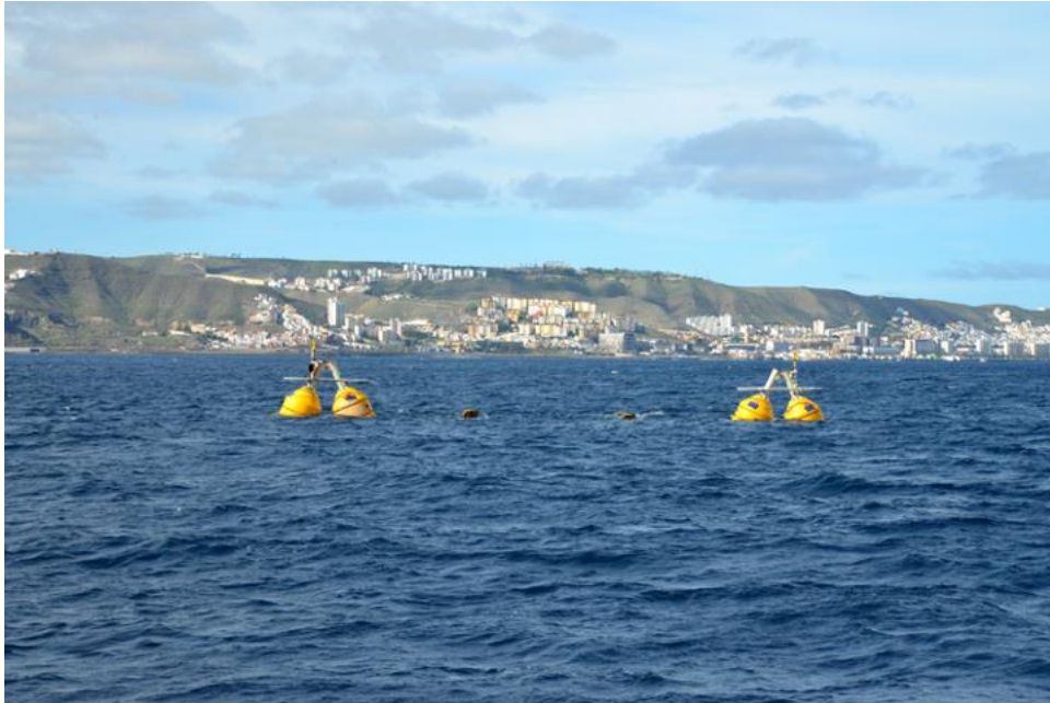
Figure 95: Wavepiston with two energy collectors operating at the PLOCAN test site.
